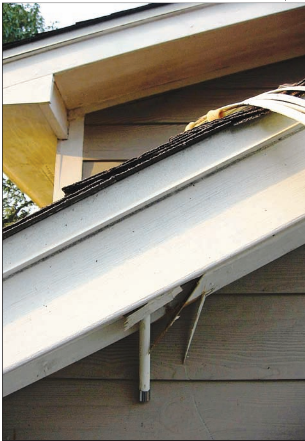
Hurricane Ike sent this Comet GP3 fiberglass vertical right through the eave.
